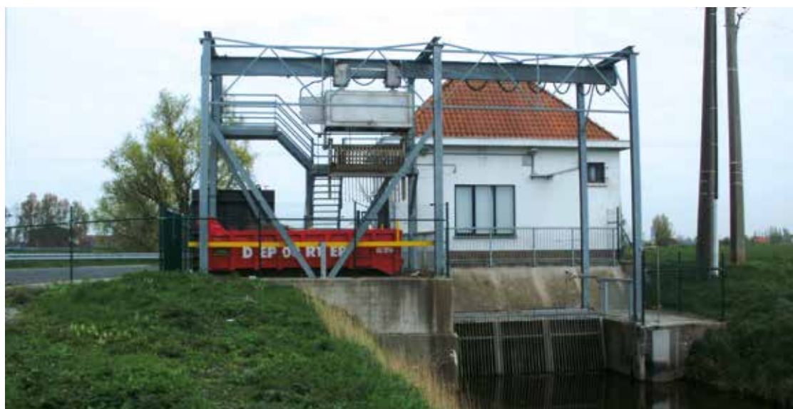
Automatic trash rack - Overhead transfer type - Woumen (Belgium)
