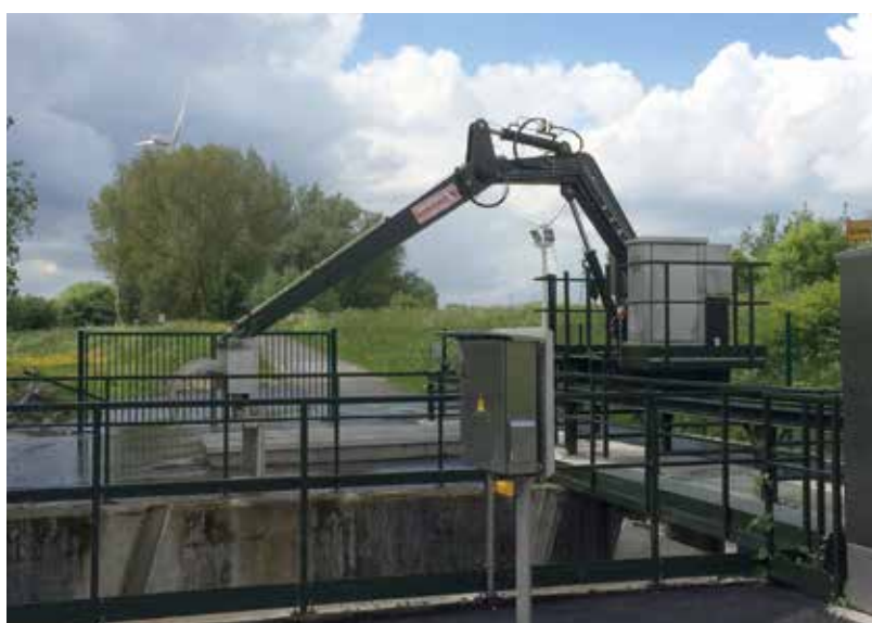
Automatic Trash Rack - Crane Type - Hemiksem (Belgium)
