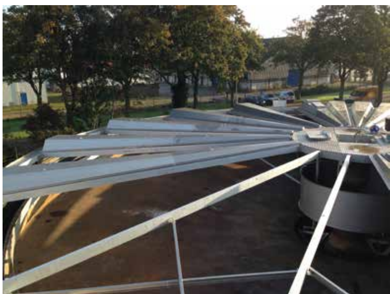
Scraper bridge with rotating roof in Aluminium - diameter tank 27 m - Dronten (Netherlands)
