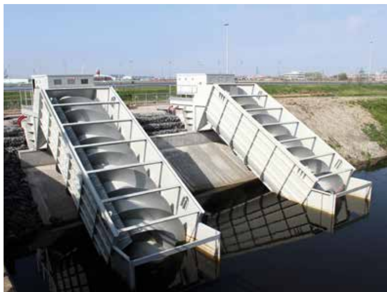
Compact screwpumps on the Leopold channel at Zeebrugge (Belgium) - 2 screws - 315 kW - 5 m 3 /s - Screw diameter 3,7 m - Bladed length 10,6 m
