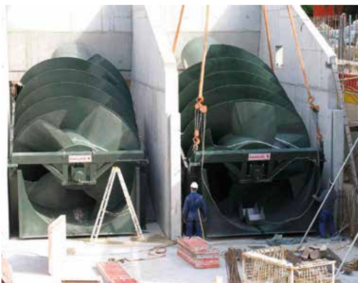
Hydro power screws with steel trough for casting at Kocherwehr Hofratsmühle in Künzelsau (Germany) - 2 screws - 132 kW - 8,95 m³/s - Screw diameter 4,1 m - Bladed length 4,8 m
