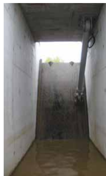
Steel construction, electromechanical and hydraulic equipment of weir at Zandvoordebrug (Belgium)
