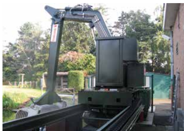
Automatic Trash Rack - Crane Type - Ertvelde (Belgium)
