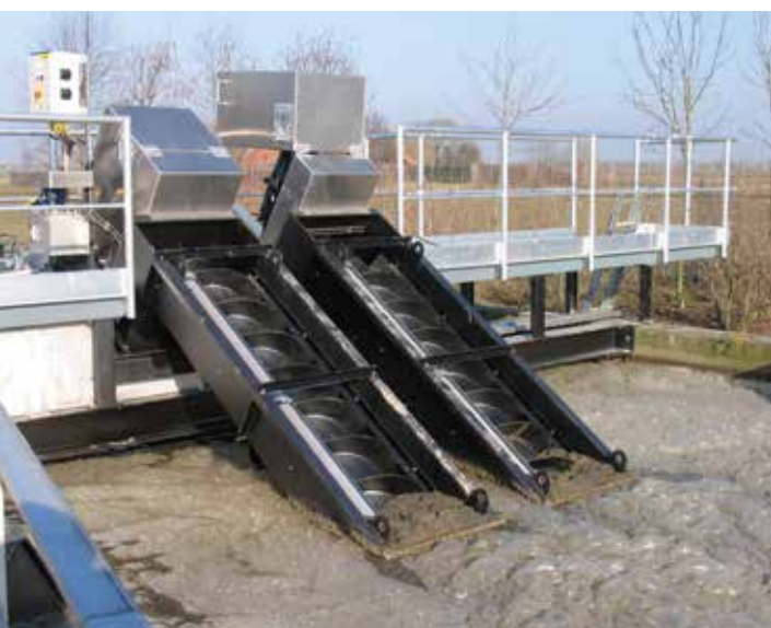
Compact screwpumps at RWZI Poperinge (Belgium)
