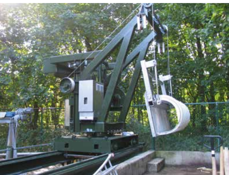
Automatic trash rack - Hybrid type - Brugge (Belgium)
