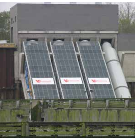
Compact screwpumps/ hydropower screws on the Albert Channel in Ham and Olen (Belgium) - 6 screws - 780 kW pumping operation - 360 kW generating operation - 5 m 3 /s - Screw diameter 4,3 m - Bladed length 21,6 m
