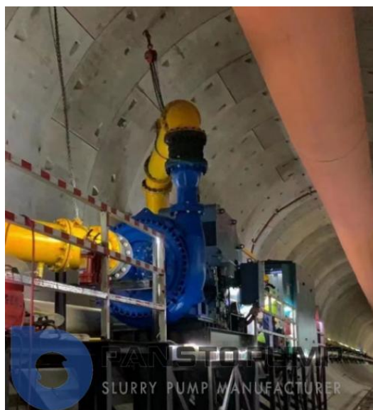
PG pumps in tunnel engineering, China
